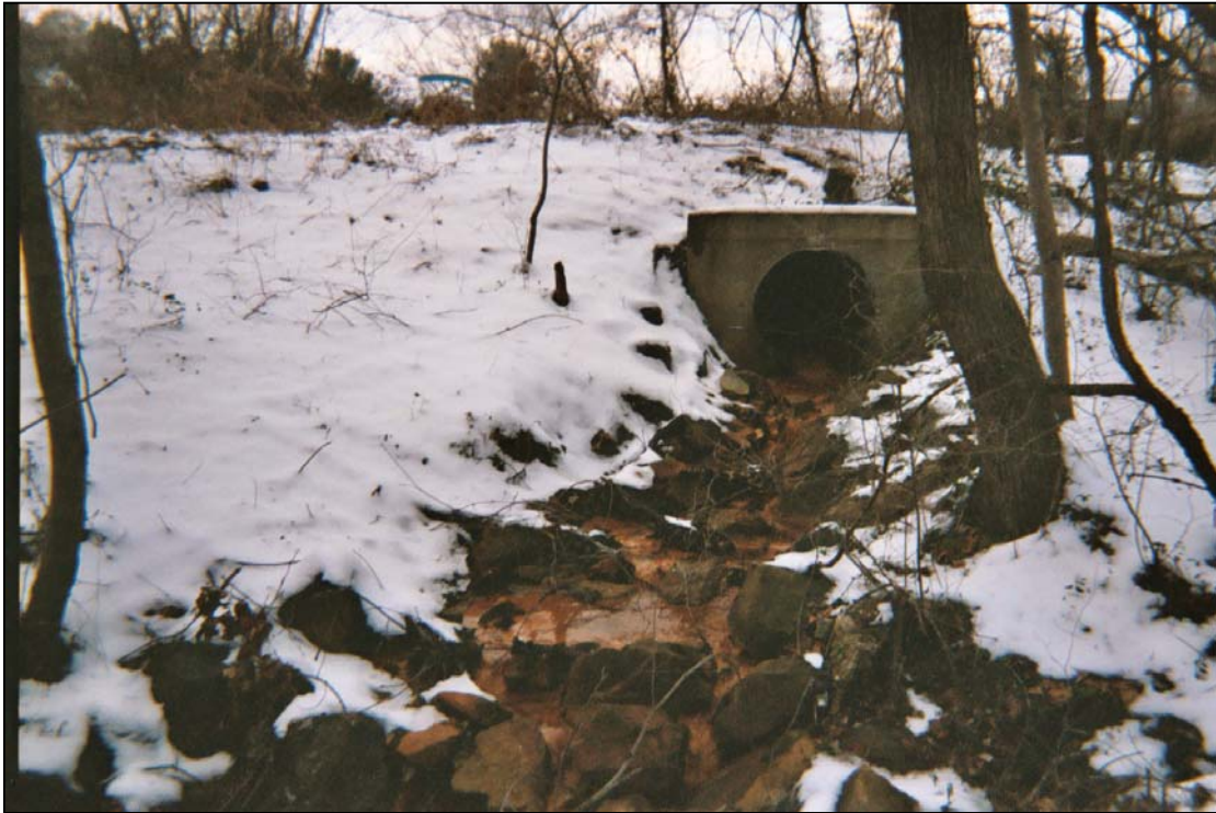
Figure 11. Hall Creek Stormwater Retrofit Opportunity
