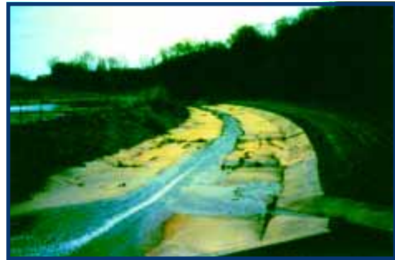
This urban stream channel has been drastically altered to increase stormwater drainage.
