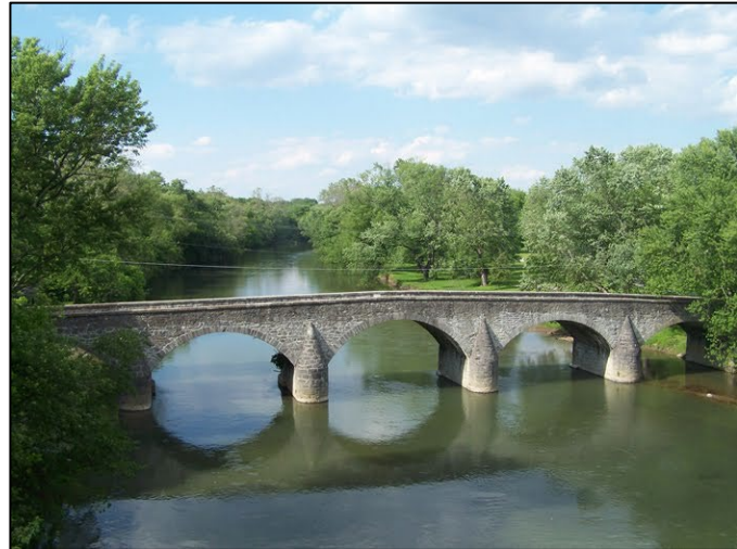
Photo 6: Wilson Bridge spanning Conococheague Creek
