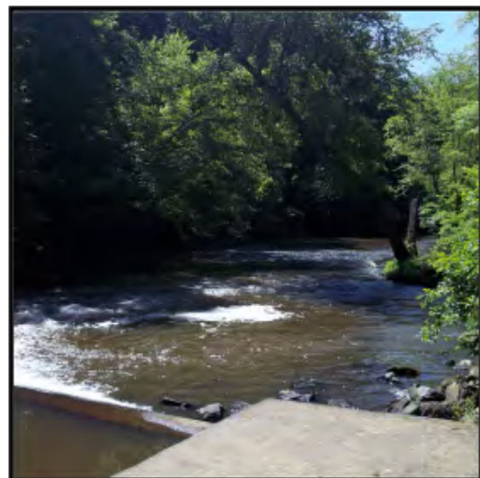
Upper Choptank USGS Spillway in the North County Regional Park, Greensboro, MD
