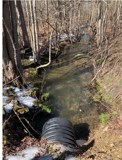
An exposed culvert at Browns Branch.
