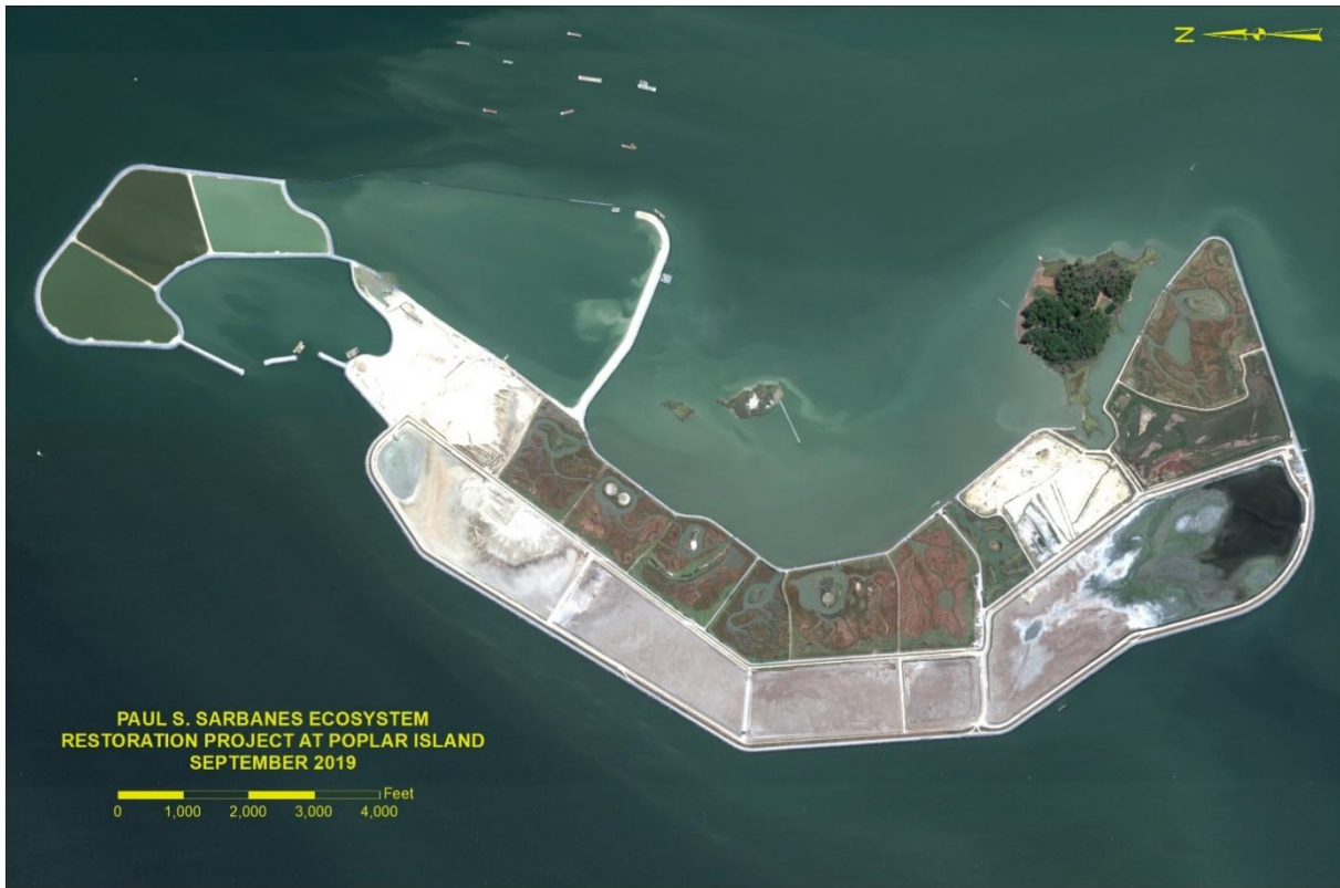
Figure 1A: Paul S. Sarbanes Ecosystem Restoration Project at Poplar Island - 2019 Aerial Photograph
