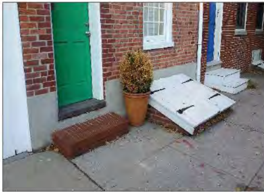
2. Foundation wall and basement access (Front)
