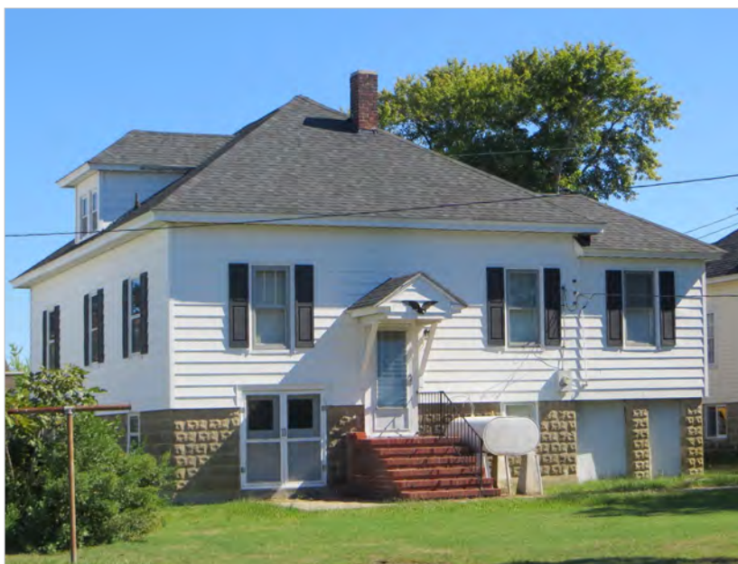
Figure 2.36 - House constructed on a higher foundation in the 1930s after an unnamed coastal storm. Ewell, Smith Island, Somerset County.
