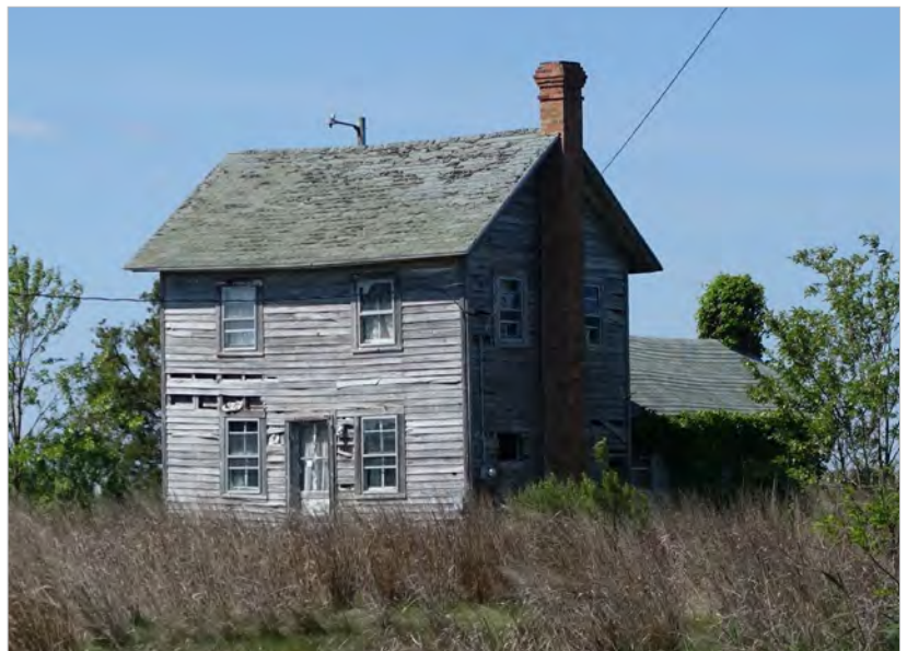
Figure 2.41 - Abandoned historic home on Hooper's Island, Dorchester County.
