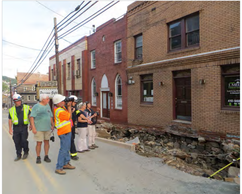
Figure 2.23 - The Maryland Historical Trust and Howard County employees conduct damage assessments after the 2016 flash flood. Ellicott City, Howard County.
