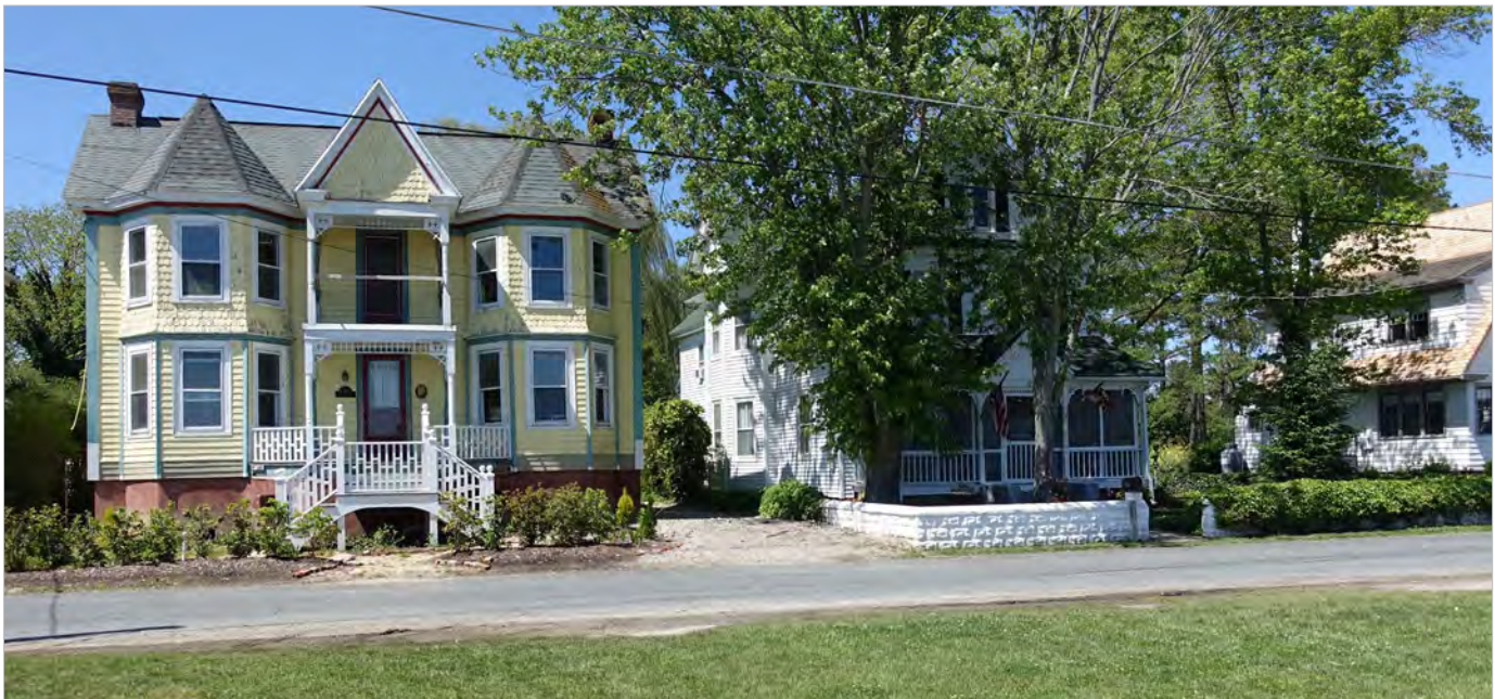
Figure 2.29 - The building on the left has been elevated, but retains its context with neighboring properties. Whitehaven, Wicomico County.
