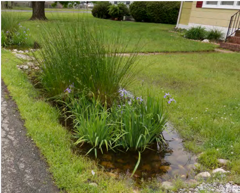
Figure 2.33 - Rain gardens provide an efficient means of minimizing stormwater runoff and can often be integrated into existing landscaping. Shady Side, Ann Arundel County.
