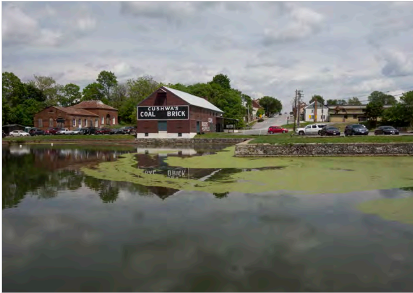
Figure 2.39 - Acceptance of building flooding: the earliest portion of this building, originally a warehouse, dates to the turn of the 19th century. The building was adapted to be a visitor center despite the risk of flooding. Flood openings are visible beneath the unpainted brick along the river-facing façade. Williamsport, Washington County.
