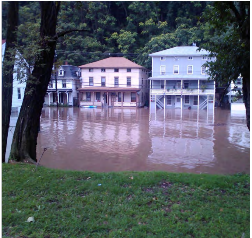
Figure 2.20 - Flooding on Main Street after Hurricane Irene, 2011. Port Deposit, Cecil County. (Source: Town of Port Deposit)
