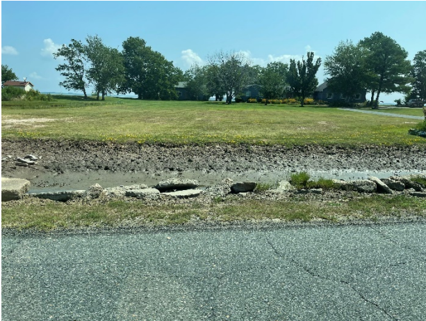
Photo 17 - Drainage Ditch along Hoopersville Road
