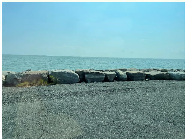
Photo 12 - Stone Revetment Protection along Road
