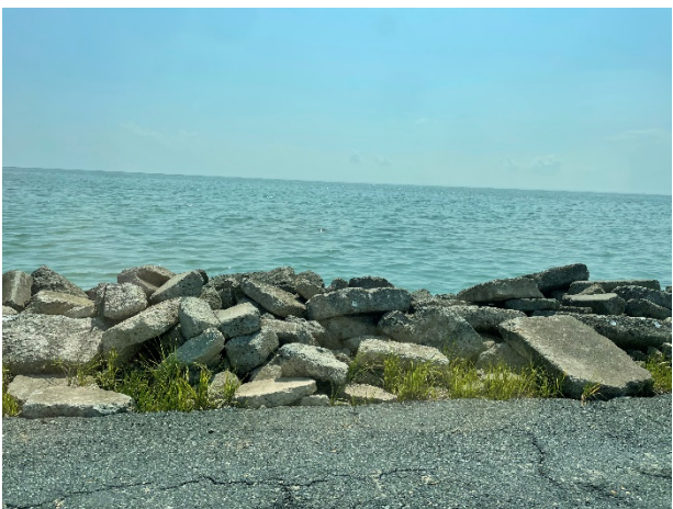
Photo 11 - Rubble Protection along Road
