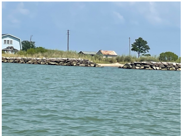
Photo 6 - Stone Breakwaters Protecting against Coastal Erosion
