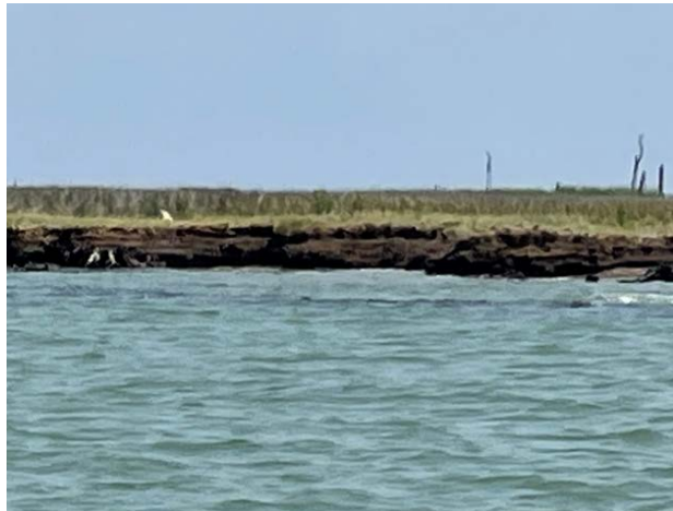
Photo 14 - Eroded Marsh Bank
