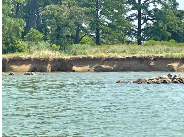
Photo 8 - Unprotected Eroded Bluff
