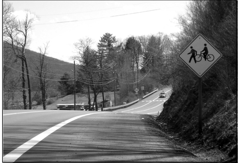
Wide shoulders and signage for bicycle/pedestrian use along US 219. Note the marked crosswalk in the background.
